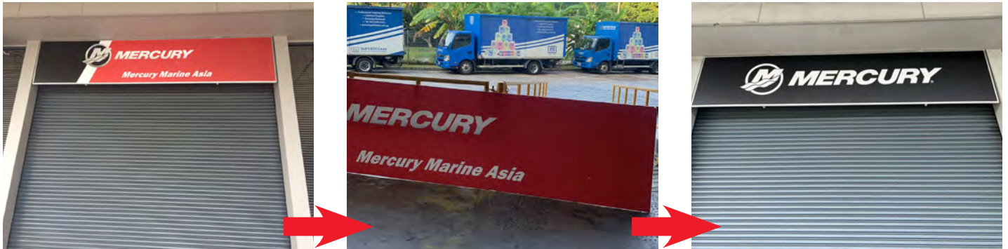
The sign above the Singapore workshop's overhead door (photo at left) was on the schedule to be updated. On the weekend before the scheduled work to replace the sign, high winds from a fierce thunderstorm pulled the sign off its mounts and deposited it against a walkway railing (center photo). Facilities workers showed up on Monday to find that the weather had accomplished the first step in the job for them.
