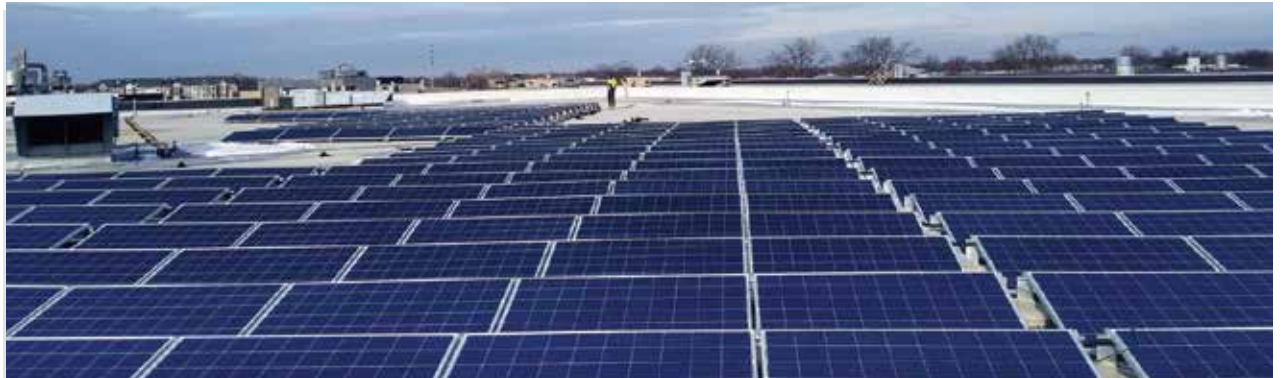
Mercury now has photovoltaic solar arrays installed at its European headquarters and its world headquarters in the U.S. The company is also included in a large-scale virtual power purchase agreement that parent company Brunswick Corporation signed in 2021.
